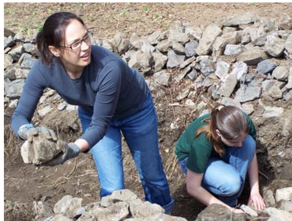
Raylene and Kathryn at work on the drainage field.
